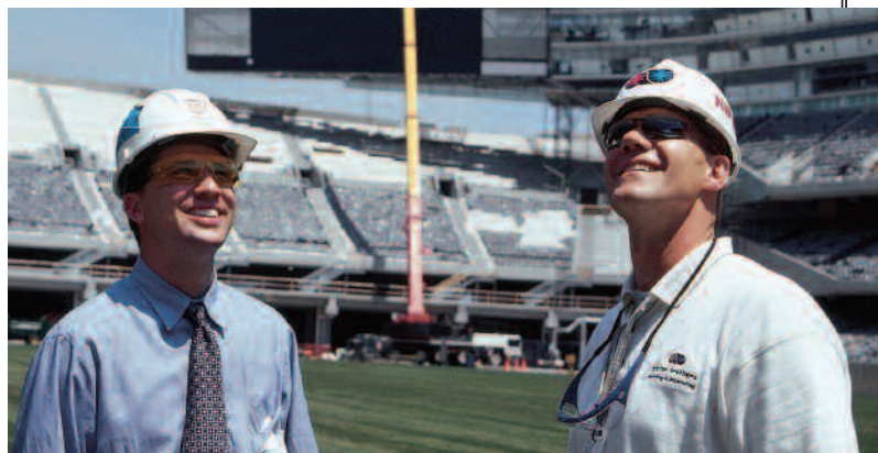
Sherwin-Williams professional coatings representative Tom Comstock (left) and Ascher Brothers Co. Inc. project manager Jim Detmer admire ongoing coatings work in Chicago.
