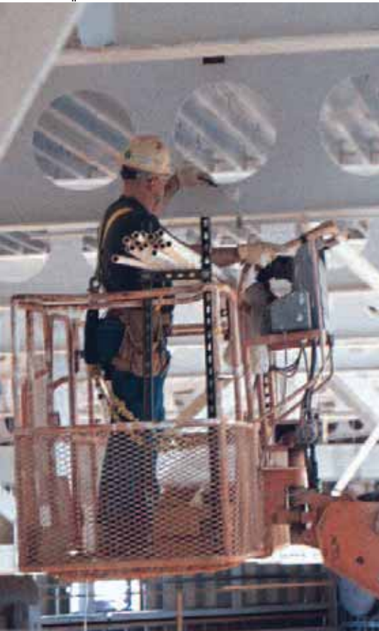
Above, touchup work occurs on some of the cellular beam work at the Opryland Hotel and Convention Center. Below, the facility rises from the Texas plain.
