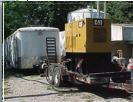
These non-potable water tanks (far left) in Frenchburg, Ky., received a FluoroKem exterior coating system, marking Caldwell's first usage of an exterior fluorourethane system.
