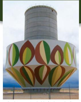
Landmark Structures' methodolgy involves performing most coatings operations at grade before the tank is hoisted to the top of the pedestal.
