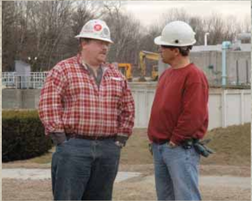
Gerry Rancourt of the Aulson Company and Bill Ouelette of Penta Construction discuss progress on the plant upgrade under way at the Merrimack (N.H.) Wastewater Treatment Plant. Below, one of the finished equalization tanks on the grounds.
